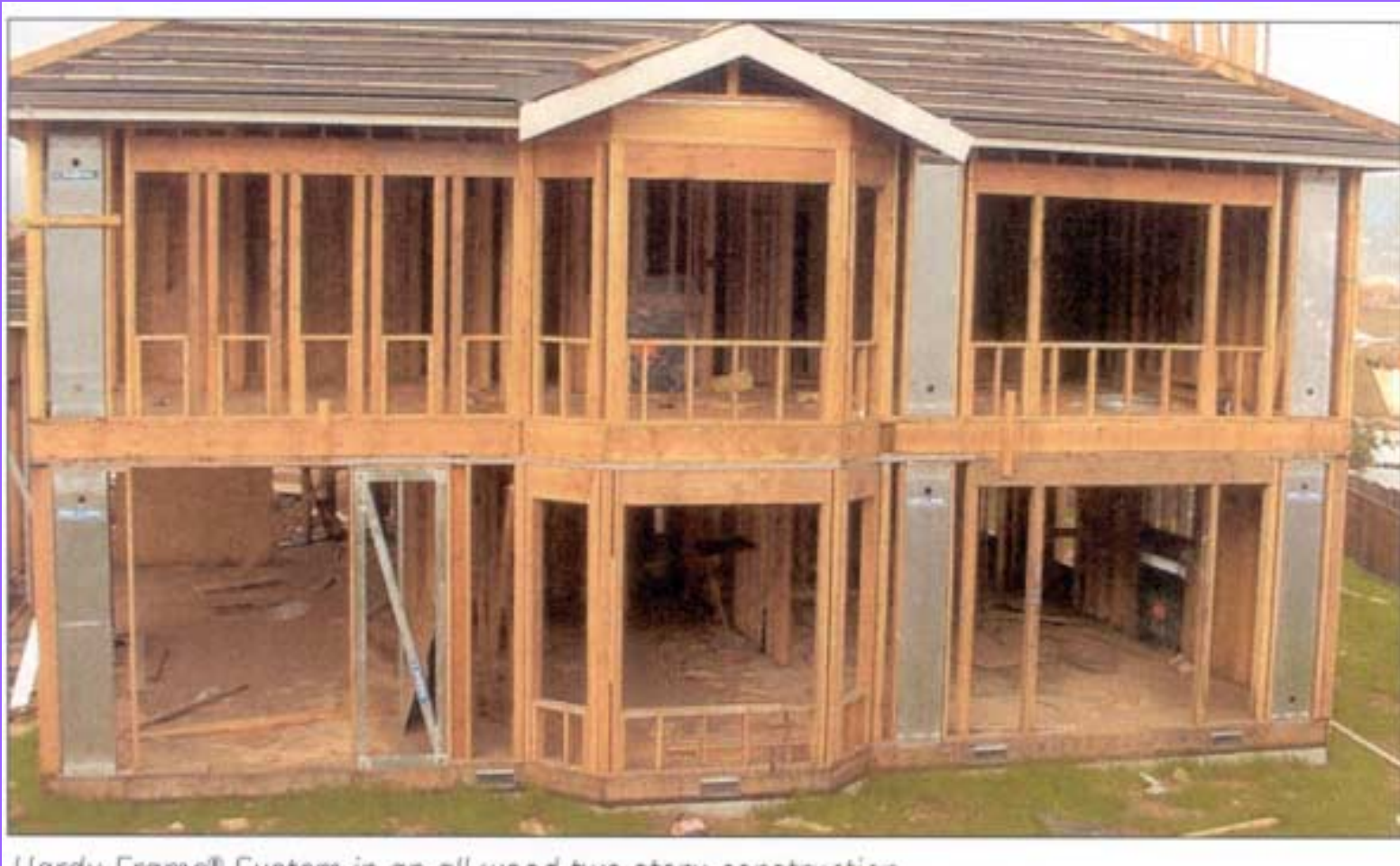
Hardy Frame® System is an all wood, two story construction
